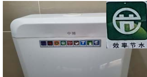
water saving toilet tank
