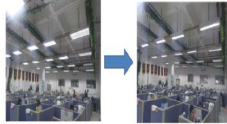
redundant lamp removal
